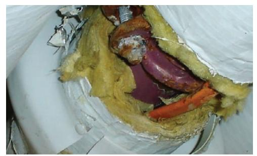
Pipe and duct corrosion is common when systems are not protected from condensation. This shortens the life of the equipment.
