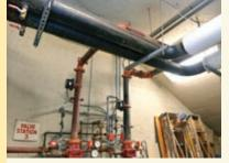
The two photos above show one set of pipes. The beautifully insulated work at the top is rendered ineffective because the insulation stops on the side of the wall not visible to the public, shown in the bottom photo.
