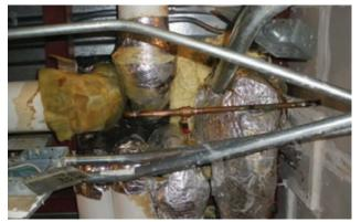
Condensation can damage concrete, ceiling tiles, drywall and wooden elements. It will also increase heat transfer rates due to the latent heat of vaporization.
