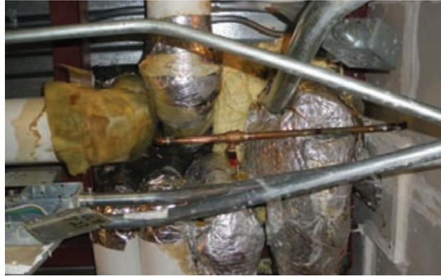
Condensation can damage concrete, ceiling tiles, drywall and wooden elements. It will also increase heat transfer rates due to the latent heat of vaporization.
