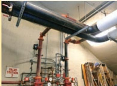
The two photos above show one set of pipes. The beautifully insulated work at the top is rendered ineffective because the insulation stops on the side of the wall not visible to the public, shown in the bottom photo.
